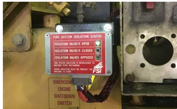
Fire System Isolation Status Panel
