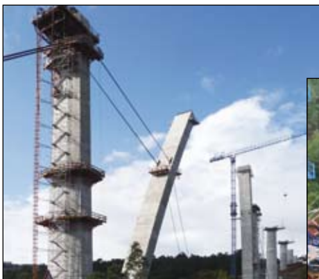
▼ Two concrete arches of this viaduct in Silleda, Spain are rotated and lowered by Enerpac Heavy Lifting Strand Jacking Systems.
